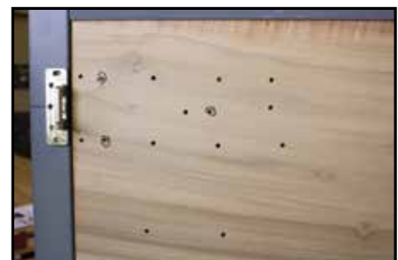
Step 11 - Fixture removed with ALL holes drilled including the optional Key Override and Wire Entry Hole
