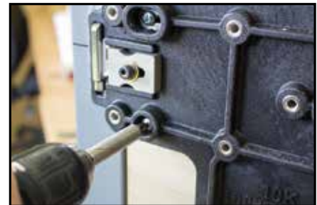
Step 9 - Once in position secure the fixture to the door with the 3 rd self tapping screw.
