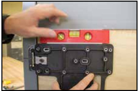
Step 4 - Align the fixture over the strike with equal clearance around the bail and level.
