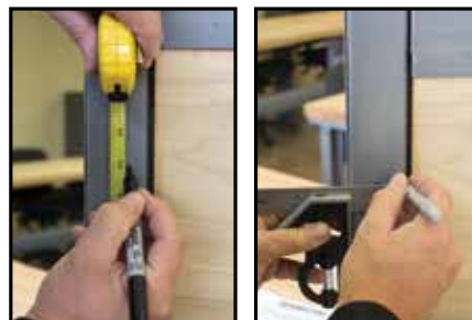
Step 1 - Measure 43" inches from the floor & mark. With a straight edge extend the mark across frame.
