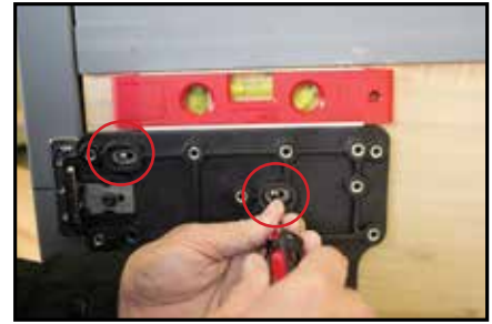
Step 7 - Level fixture to the door and secure with (2) self tapping screws into the slotted mounting holes.
