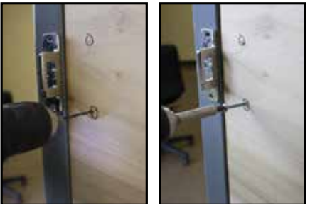
Step 6 - Drill pilot holes for the (3) mounting holes and pre-thread the holes with the provided screws.
