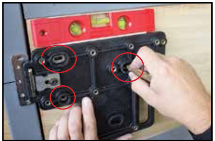
Step 5 - Once in position and level, center punch the (3) mounting holes (see circled areas above)
